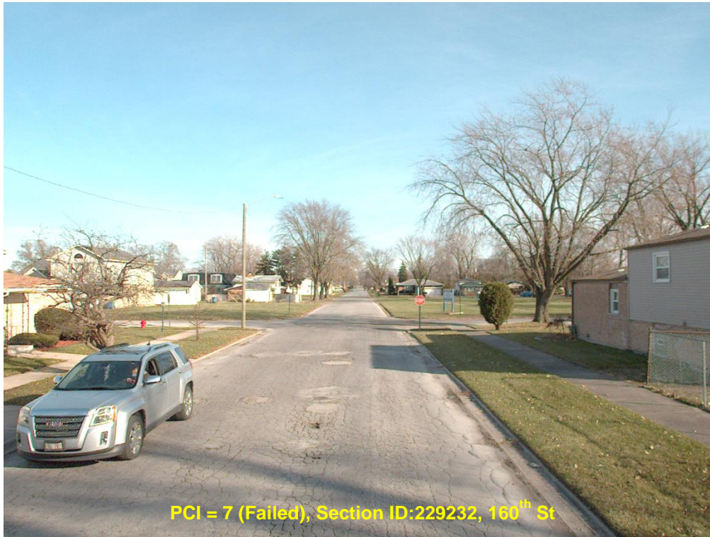
Figure 8: Sample pavement image with 'Failed' PCI value.
