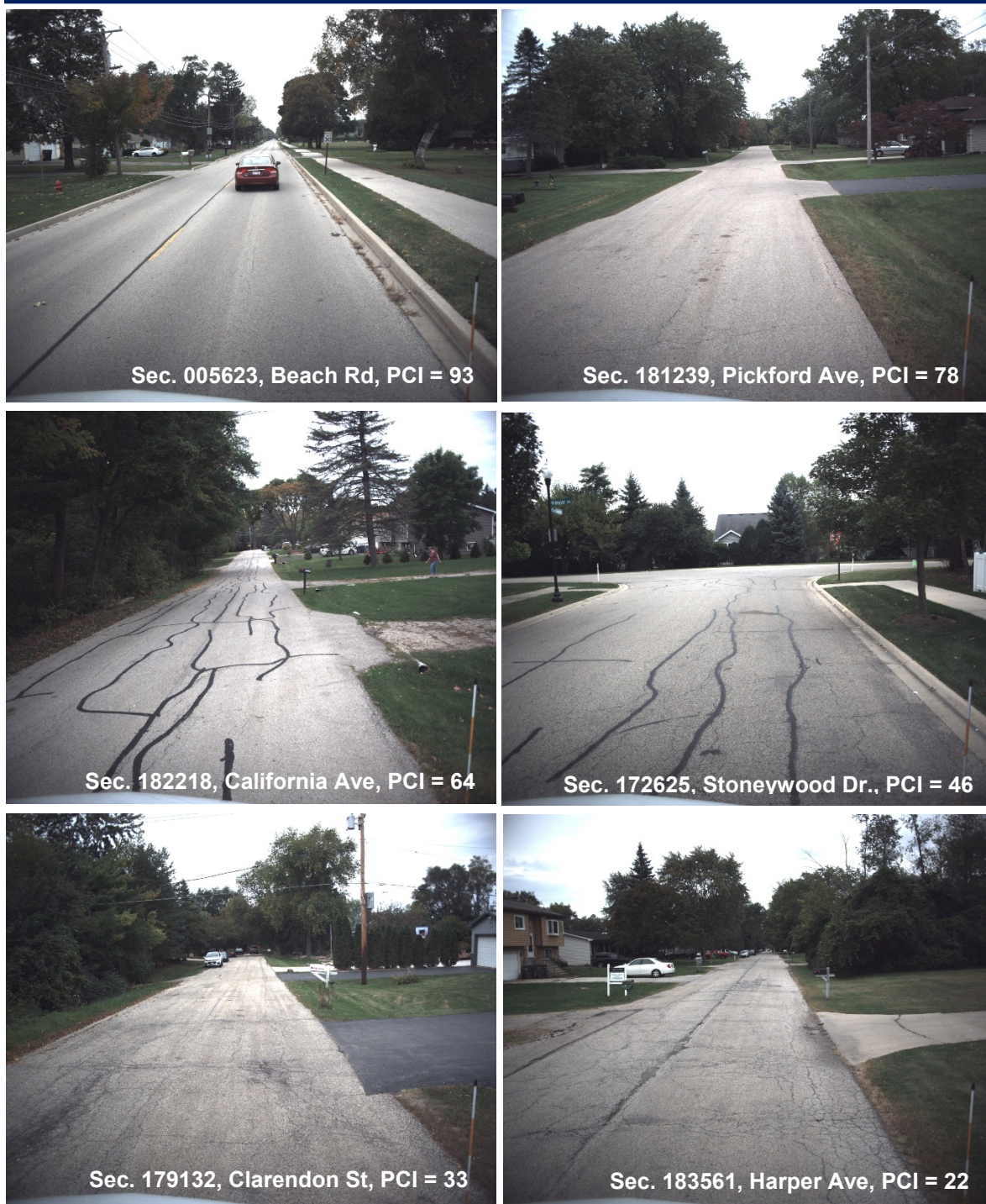
Figure 7. Sample pavement images with different PCI values (Good-Serious).
