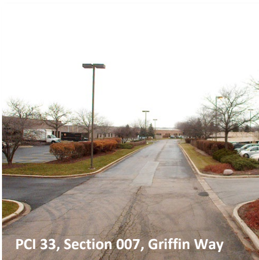
Figure 7. Sample pavement images with different PCI values.
