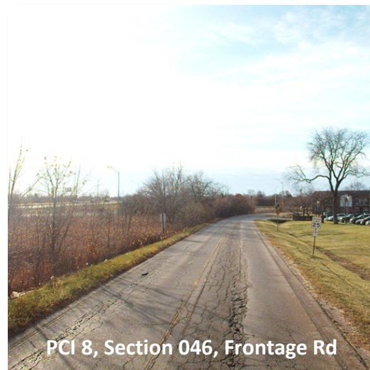
Figure 7. Sample pavement images with different PCI values.
