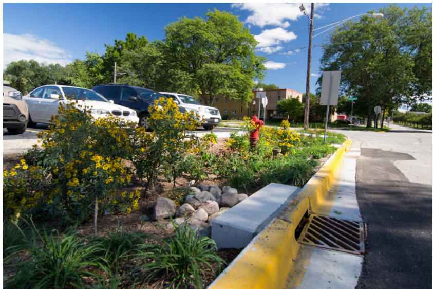
A series of rain gardens helps with surface runoff from the parking lot of Holy Angels in Aurora, IL. Source: RainReady: Center for Neighborhood Technology, 2017.
