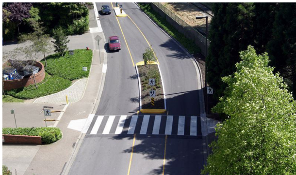
High-visibility crosswalks typically make use of longitudinal or “continental” pavement markings, which are highly visible to approaching traffic.
