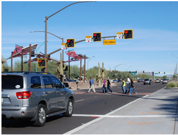
Pedestrian-activated hybrid beacons, such as the example pictured above, facilitate safe mid-block crossings and uncontrolled intersections.
