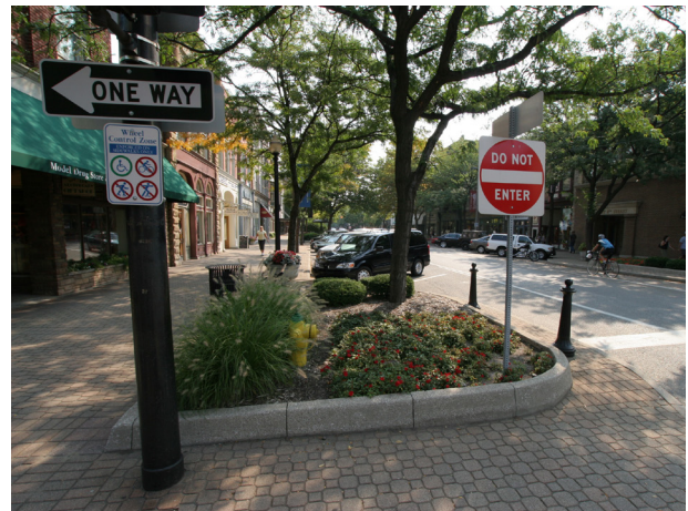
Street trees and bump-outs, such as the example pictured above, can enhance the atmosphere of the streetscape and entice people to walk, and have been shown to produce economic benefits for properties nearby.
