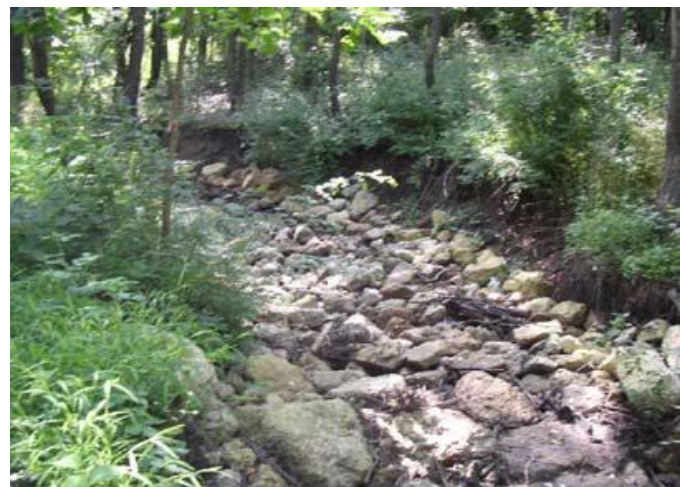
Bend reconfigured, graded, and rock riffles installed
