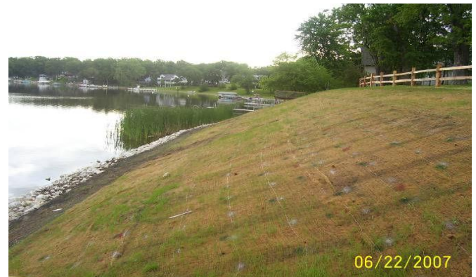
Post-construction shoreline conditions
