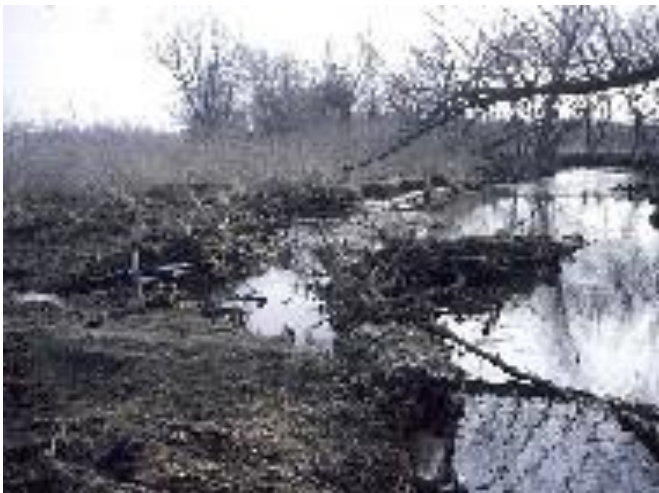
Pre-construction conditions, blowout area from upstream showing sediment
