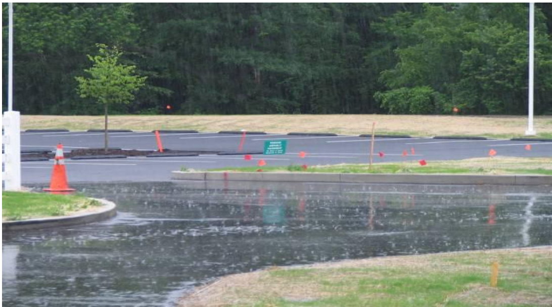
Rain falling on a conventional street surface (foreground) and generating stormwater runoff, a significant contributor to non point source pollution, next to a new porous-pavement parking lot (background) doing its job of preventing stormwater runoff that is typically associated with impervious surfaces (photo courtesy of Lake County Forest Preserves District).
