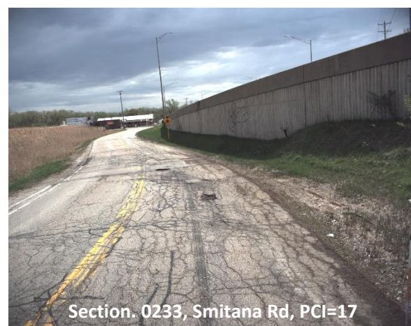
Figure 7. Sample pavement images with different PCI values.
