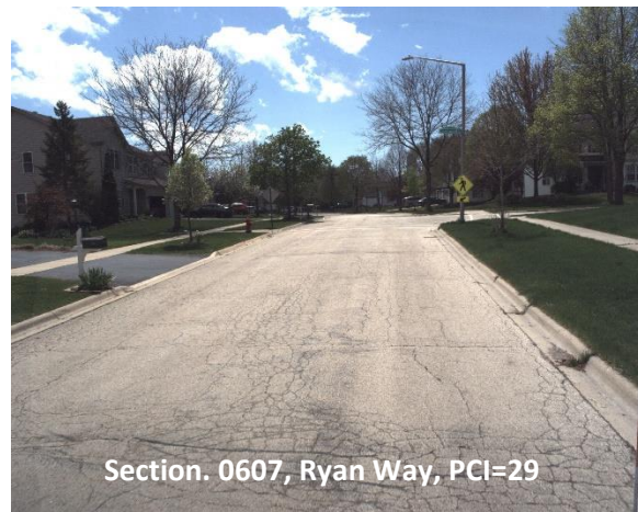
Figure 7. Sample pavement images with different PCI values.
