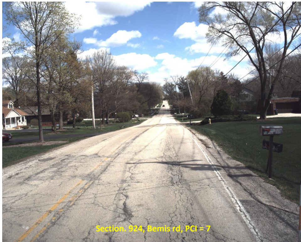
Figure 8: Sample pavement image with ‘Failed’ PCI value.
