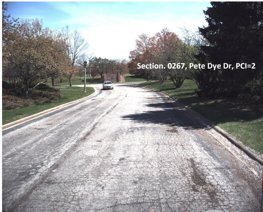
Figure 8. Sample pavement image with ‘Failed’ PCI value.
