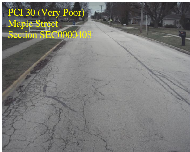
Figure 8. Example street segments at different PCIs.
