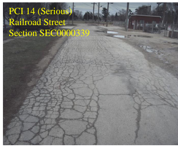
Figure 8. Example street segments at different PCIs.
