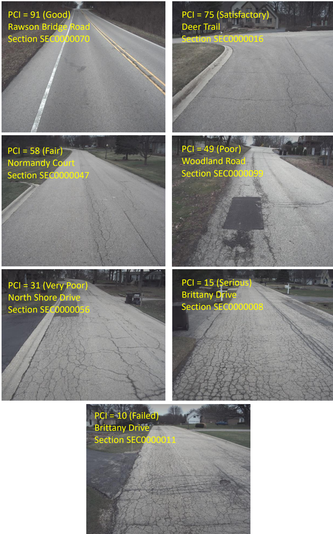
Figure 7. Example street segments at different PCIs.
