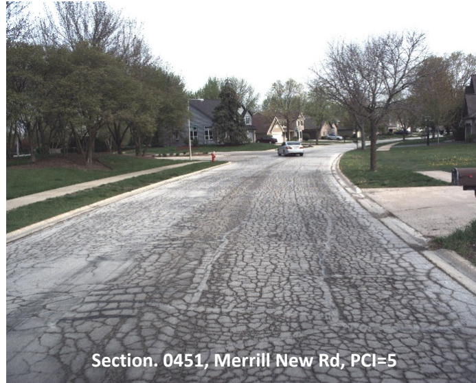
Figure 8. Sample pavement images with ‘Failed’ PCI value.
