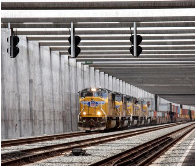
Figure 1. Alameda Corridor project
