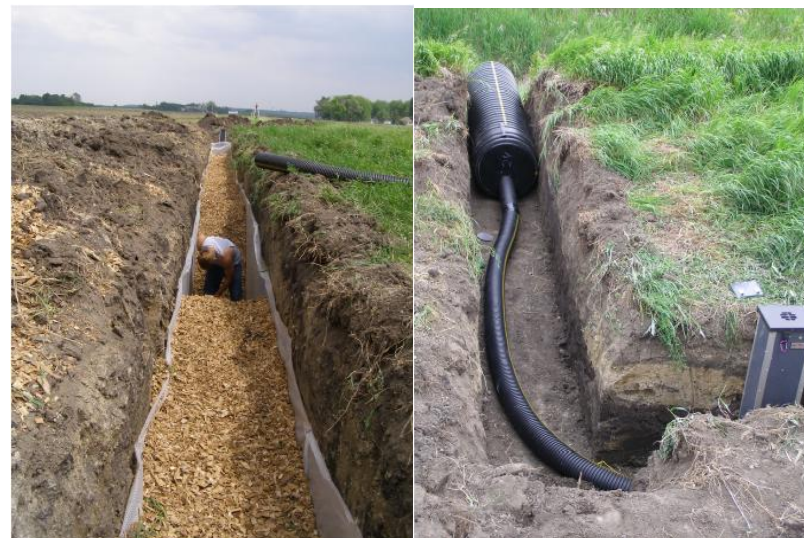
Figure 5-5. Installation of a woodchip bioreactor.
