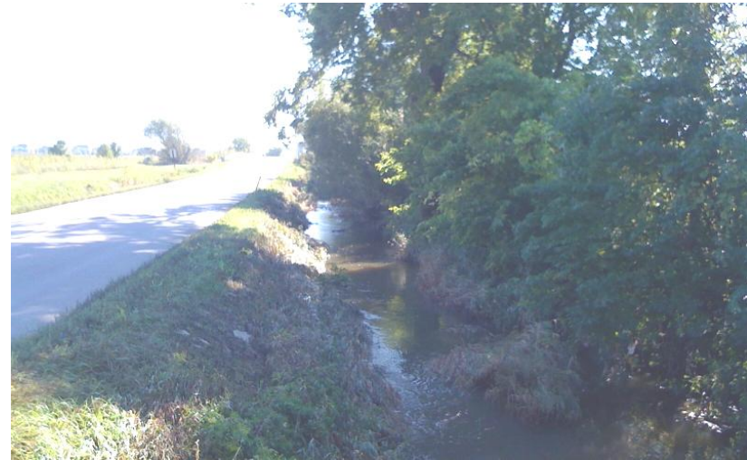
Figure 2-20. Section of Jackson Creek in Frankfort to be remeandered (near intersection of 116 th and Steger)
