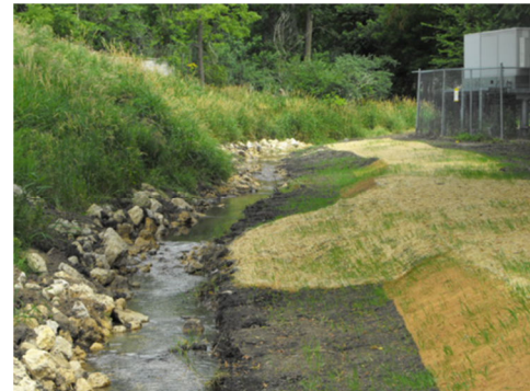
Figure 4.9 Example streambank stabilization project.
