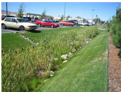
Figure 4.2 Vegetated swale. (Source: werf.org)
