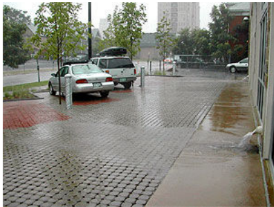
Figure 4.8 Example permeable pavement.
