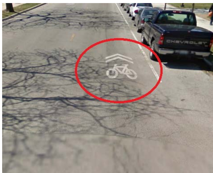
Figure 2.3: 33 rd Street shared lane identifier
