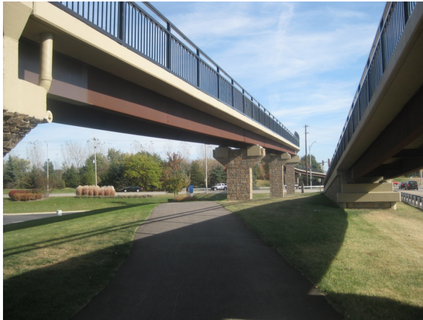
Figure 2.6: Pedestrian bridge over Randall Road, St. Charles
