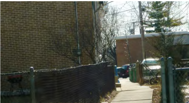
Figure 3.45: No lighting along the walking path makes this secluded area a more likely location for crime, or at least an unsafe feeling, after dark. Cars parked at both ends of the sidewalk also block view of any activity within this area.
