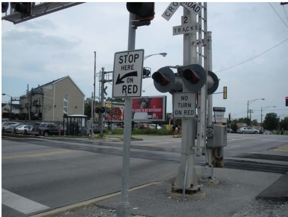
Figure 2. Crossing 608830M – A view from the ground.
