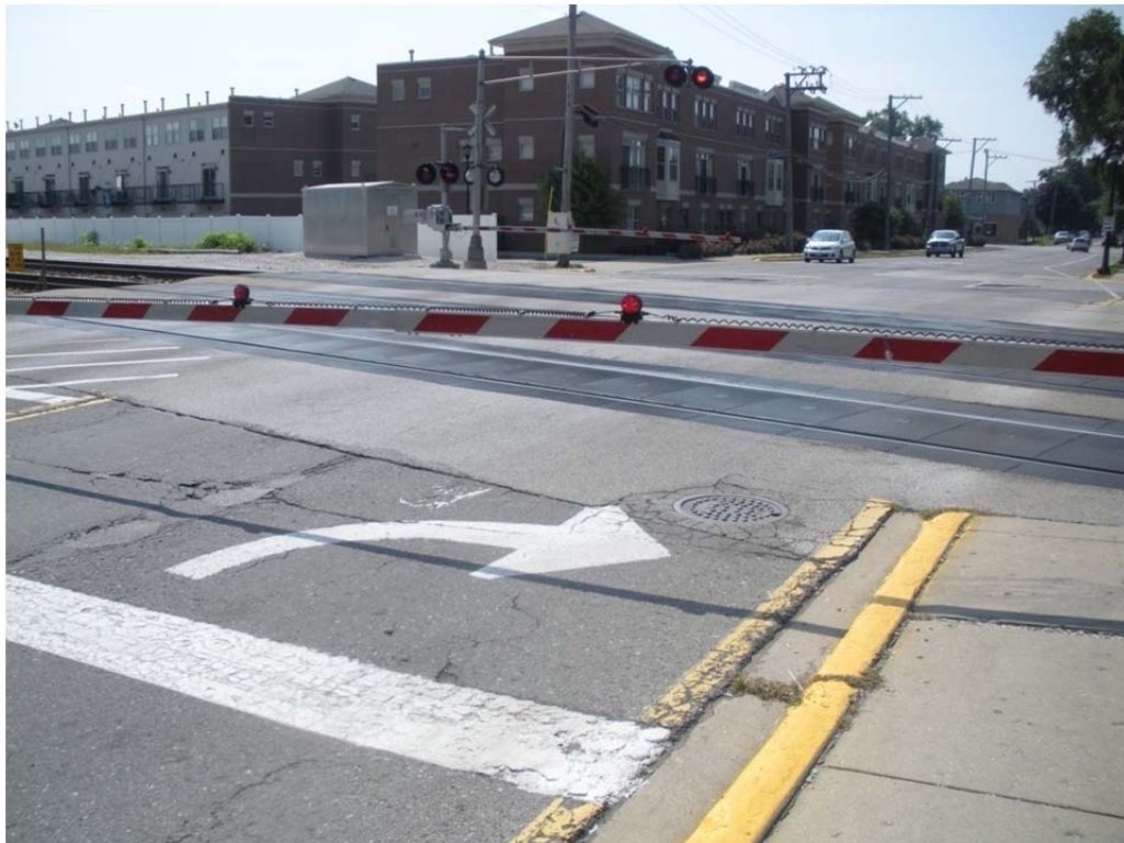
Figure 20. Crossing 372128W – A view from the ground.
