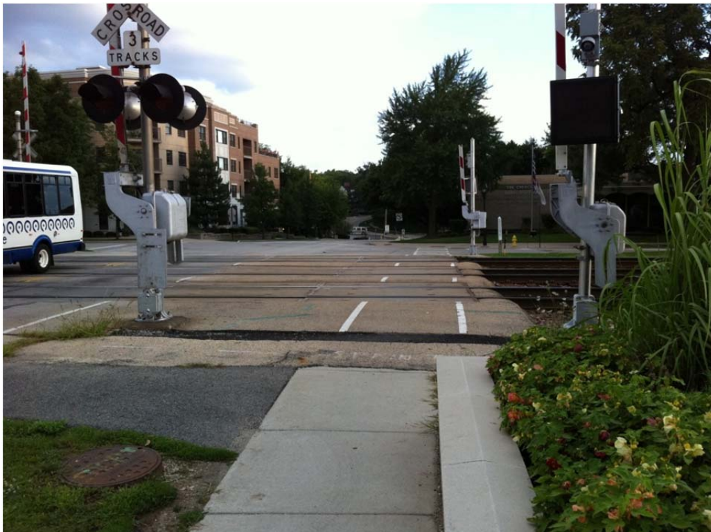
Figure 10. Crossing 174948Y – A view from the ground.
