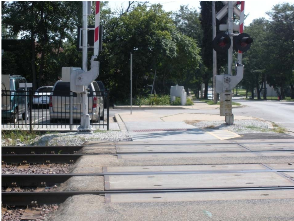
Figure 18. Crossing 174937L – A view from the ground.
