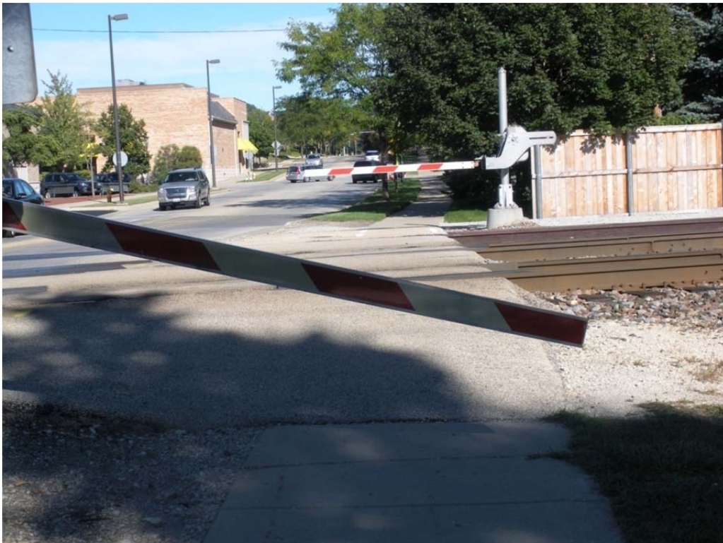
Figure 14. Crossing 388040W – A view from the ground.
