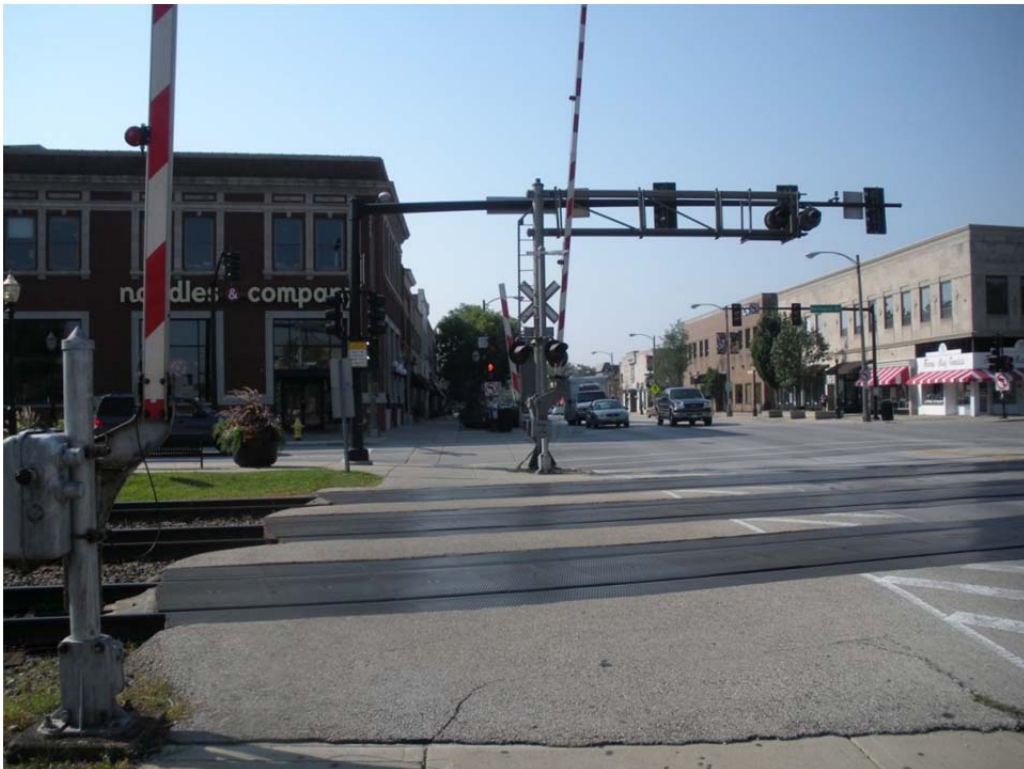
Figure 8. Crossing 079508Y – A view from the ground.
