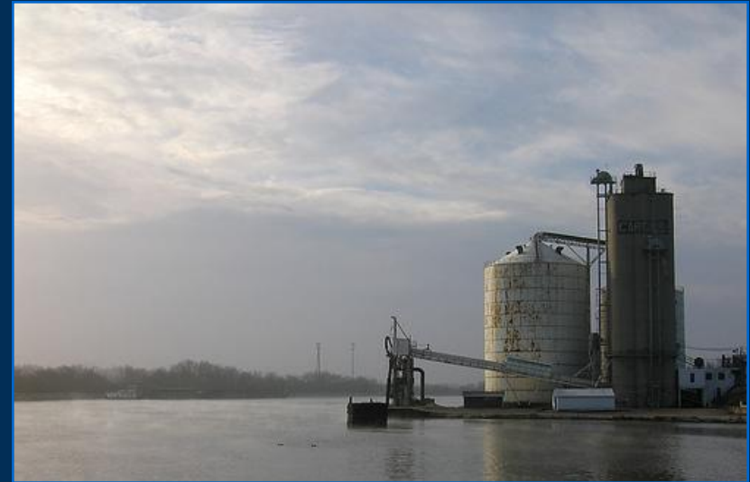
Grain Silo in Lockport on Illinois River (Jim Frazier)
