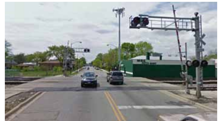
71 st Street Highway Rail-Grade Crossing
