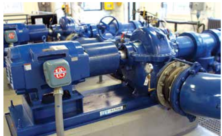
Variable Speed Pumps at the Oak Park Central Pumping Station. Source: Oak Park.
