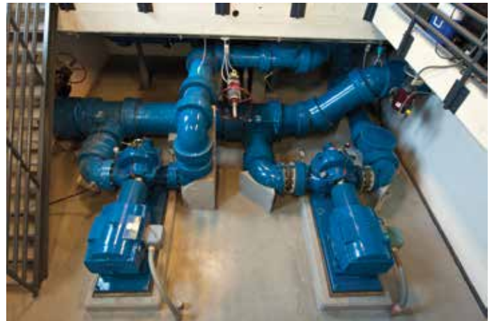
Variable Speed Pumps; Used for soft start and stops reducing water hammer and consistent flows and pressures. Source: Oak Park.
