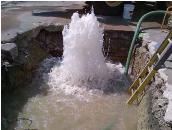
Aging Infrastructure; Oak Park water main break on a 20-inch water main. Source: Oak Park.
