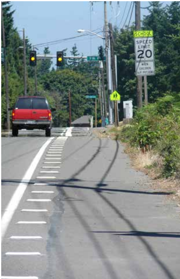
Figure 72. Wide paved shoulder can accommodate bicycle travel in rural areas
