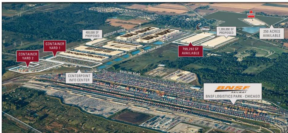
Figure 21. Aerial view of CenterPoint Logistics Park in Elwood, IL
