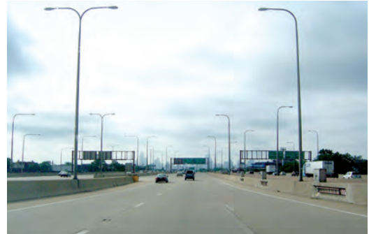
Managed lanes such as express lanes and reversible lanes separate vehicles by trip destination and by vehicle type. Conflicts and weaving are minimized; capacity is optimized. Structural barriers are the primary means of assuring optimum system performance. In Chicago, IDOT maintains the reversible lanes on I-94, at the junction with I-90 to south of the loop. These lanes are switched during rush hour to mitigate peak demand periods. Express lane facilities typically serve passenger cars only and provide point-to-point service with a much lower frequency of access and egress points. Photo by Flickr user HelveticaFanatic
