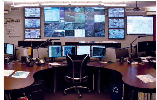
Lake County’s “Program for Arterial Signal Synchronization and Travel Guidance” (PASSAGE) gives motorists real-time information about traffic bottlenecks via electronic signs or an AM radio station. Based on the same information collected by cameras and traffic sensors, operators can also adjust traffic signal timing to reduce congestion buildup. This still-expanding ITS system is a model for other counties. Image courtesy of Lake County
