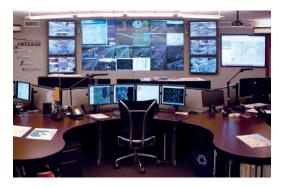
Lake County's "Program for Arterial Signal Synchronization and Travel Guidance" (PASSAGE) gives motorists real-time information about traffic bottlenecks via electronic signs or an AM radio station. Based on the same information collected by cameras and traffic sensors, operators can also adjust traffic signal timing to reduce congestion buildup. This still-expanding ITS system is a model for other counties. Image courtesy of <u>Lake County</u>
