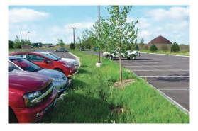
Among other stormwater best management practices, the Lake County Central Permit Facility uses native plant bioswales. These shallow excavated swales with deep-rooted native plants are designed to collect, absorb, and filter stormwater runoff and pollutants that collect on the parking lot pavement from automobiles. County government can be a leader in using stormwater best management practices. Photo and description courtesy of Lake County.
