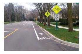
In Wilmette, an 18-month construction project has converted 4-lane Sheridan Road into a 2-lane road with bike lanes in either direction and a middle turn lane from Lake Avenue north to Westerfield Drive and the Plaza del Lago. Image courtesy of the <u>Village of Wilmette</u>
