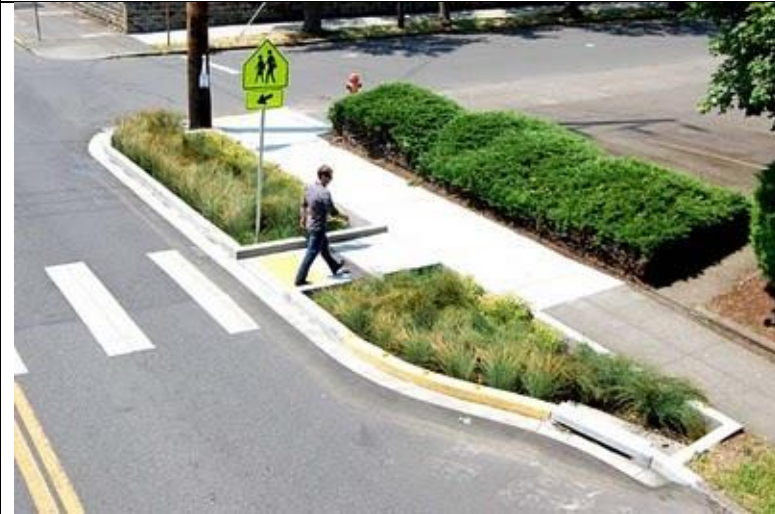
Figure 5.4: Curb Extensions with Green Infrastructure
