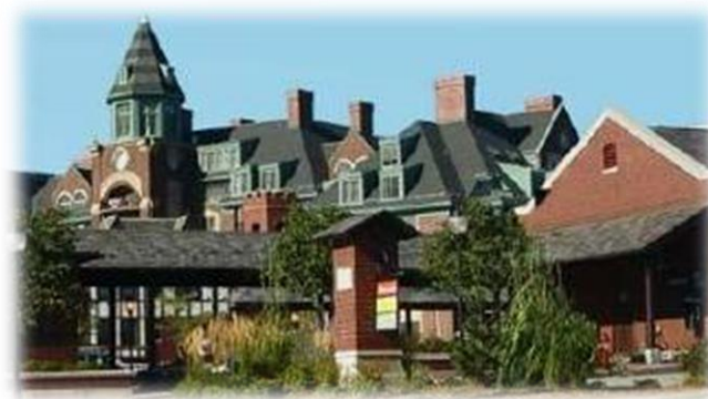
Village Green and Train Station Source: Village of Arlington Heights and Calder Latour
