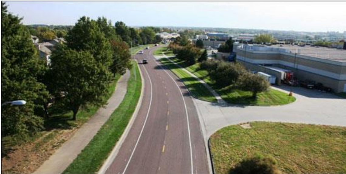
Bike lanes were added to 133rd Street in Overland Park, KS, by narrowing excessively wide lanes. Bike lane markings and signs had not yet been installed when this photo was taken. Photo credit: John Keating, City of Overland Park, KS.
