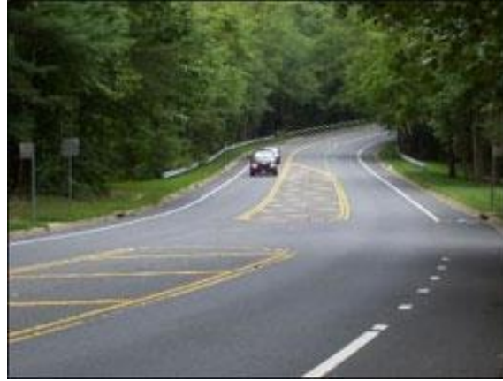
Bike lanes were added to Soapstone Dr. in Reston, VA, through a Road Diet. Credit: R.Dittberner, Virginia DOT
