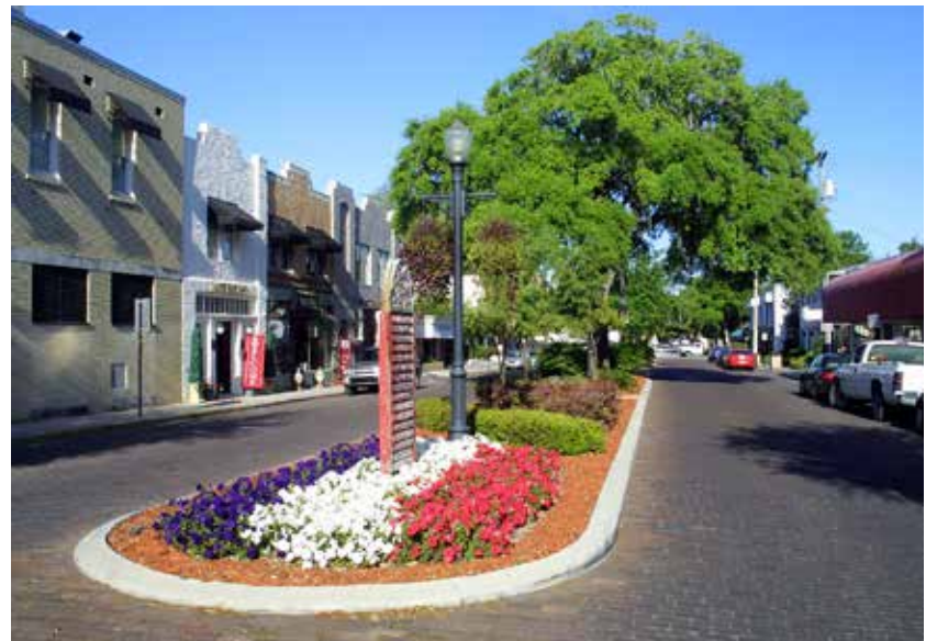
A pedestrian refuge and planted median (top) and local gateway feature (bottom) should be considered for inclusion in future reconfiguration of the IL Route 53 right-of-way. Photo Credit: Dan Burden.
