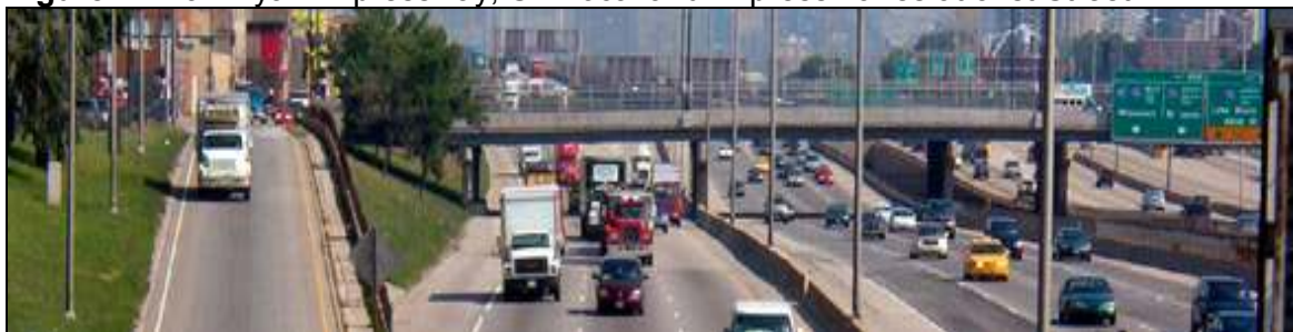
Figure 1. Dan Ryan Expressway, SB Local and Express Lanes at 31st Street
