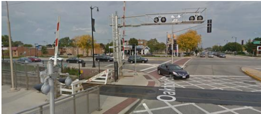
Remove right-turn lane/pork chop, change to no turn on red, and/or add a speed table/elevated crosswalk
