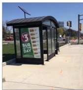
Bus and Rail Warming Shelters
