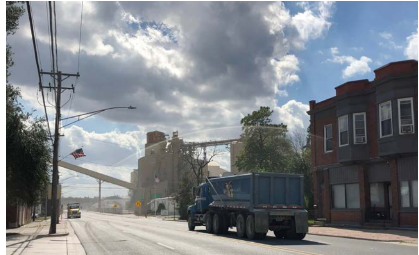
Williams Street looking south at Hanson aggregate facility.
