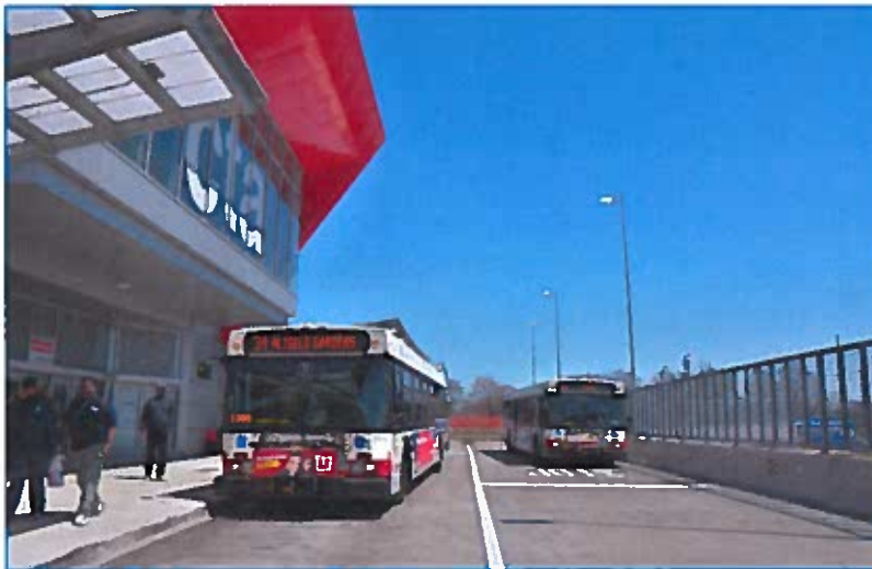
CTA's #34 South Michigan bus picking up passengers at the 95 th /Dan Ryan station. The Red Line Extension will provide increase accessibility to homes and jobs for passengers headed south of the 95 th /Dan Ryan station.
