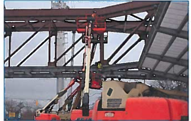
Construction workers completing improvements at the 95 th /Dan Ryan Station.
