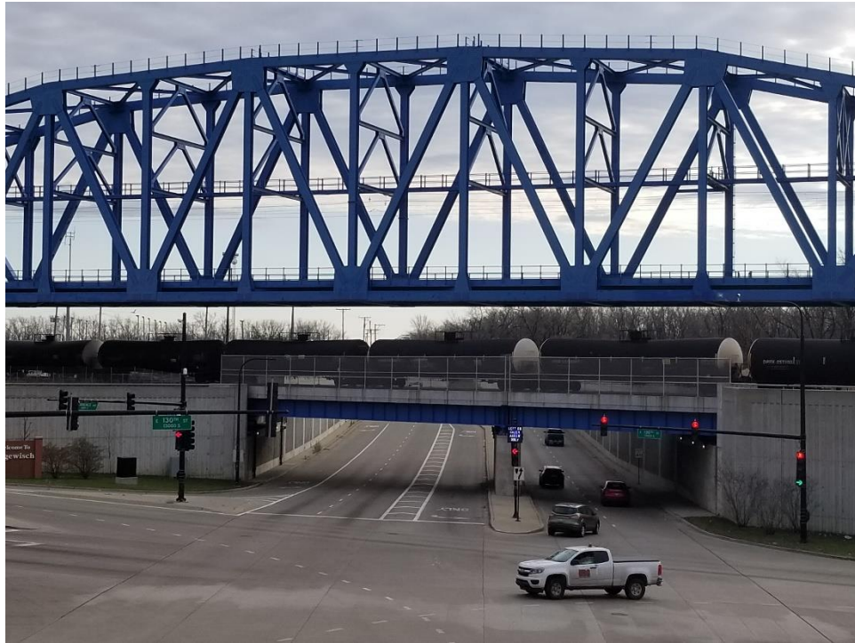
130 th St at Torrence Ave, Chicago
