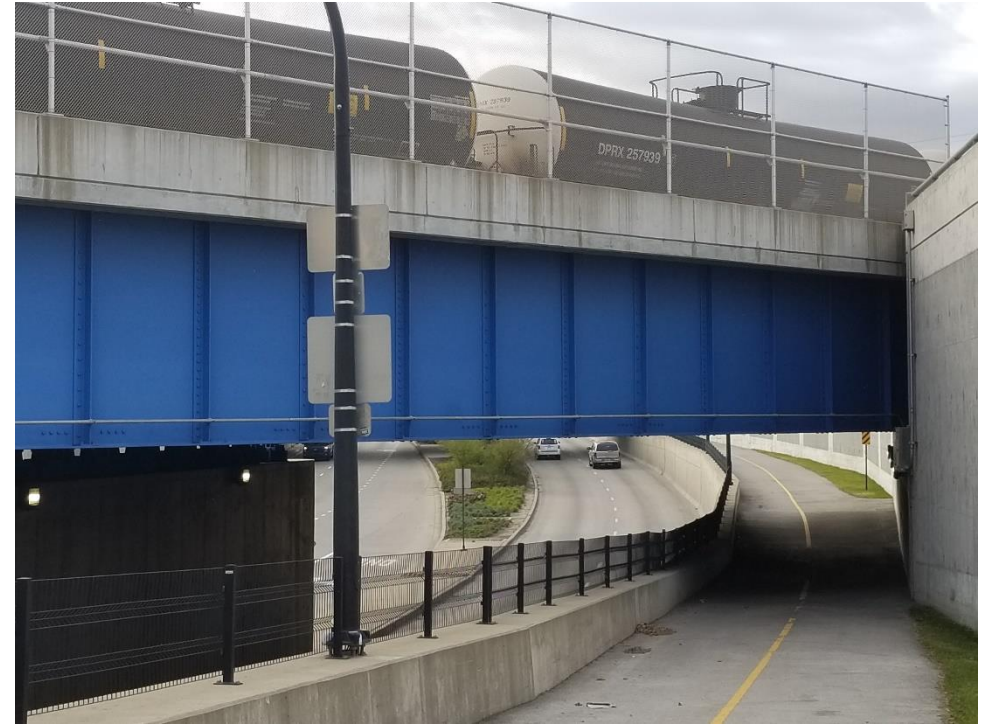
130 th St at Torrence Ave, Chicago
