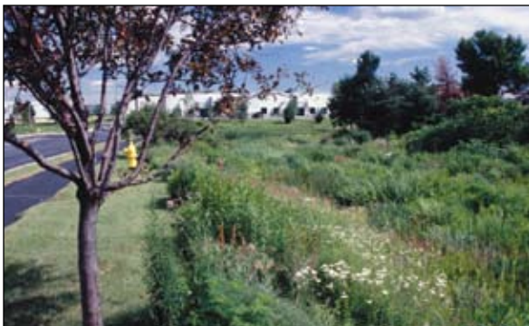
Drainage swales, planted with native vegetation can reduce both the volume and rate of stormwater runoff (Tellabs Company, Naperville, Illinois).
