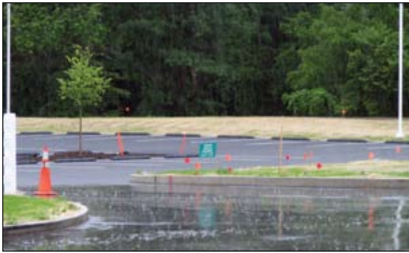
Porous Pavement Example 1: Porous pavement (background) parking lot, adjacent to conventional street during rain storm at Ryerson Woods Welcome Center. Porous pavement allows infiltration and reduces runoff (Lake County, Illinois).
