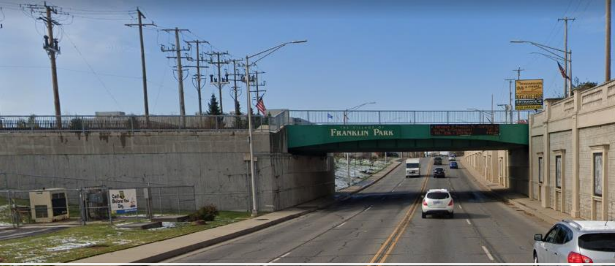
Example – Hwy/Rail Grade Separations
