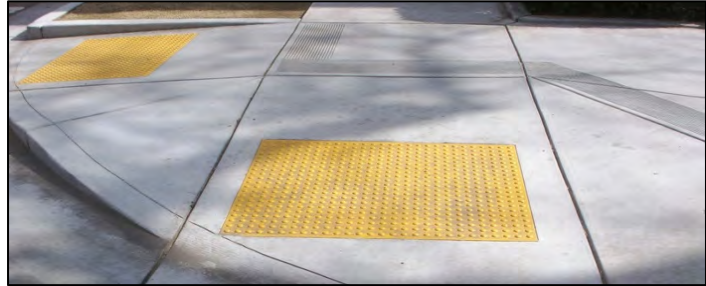
Figure 5-17. ADA-compliant sidewalk curb ramps
