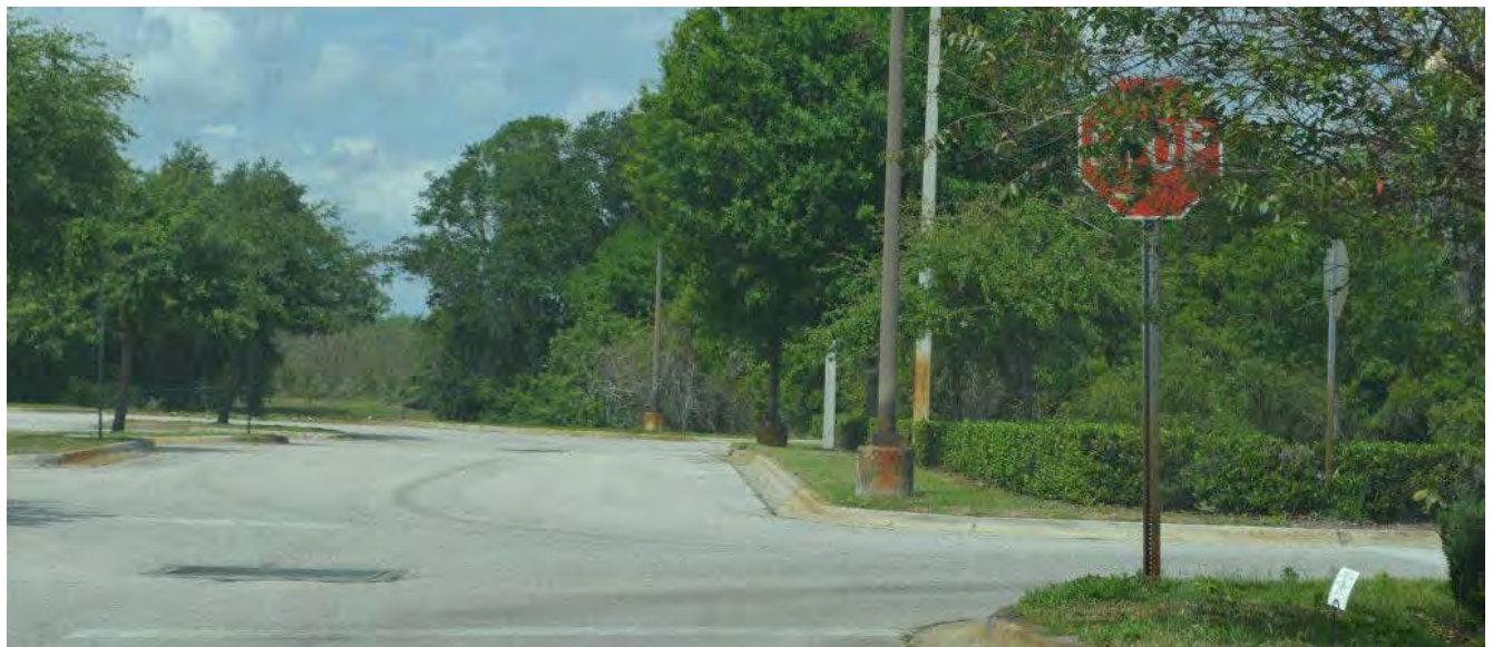
Figure 3-19 Stop sign blocked by tree ( source )
