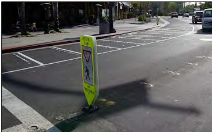
Figure 5-34. In-street pedestrian crossing sign
