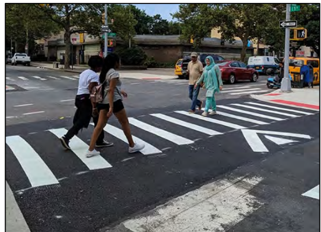
Figure 5-23. Raised crosswalk example
