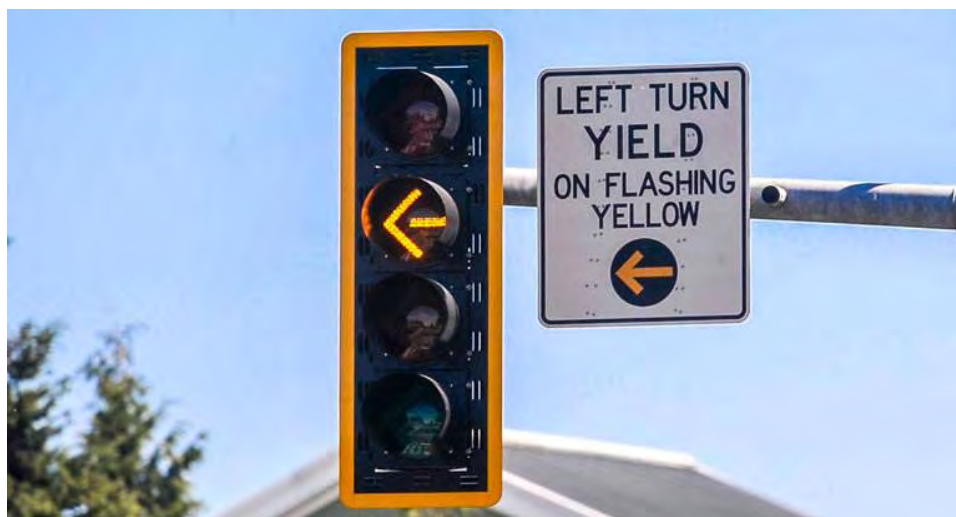
Figure 3-15 Flashing yellow arrow ( source )
