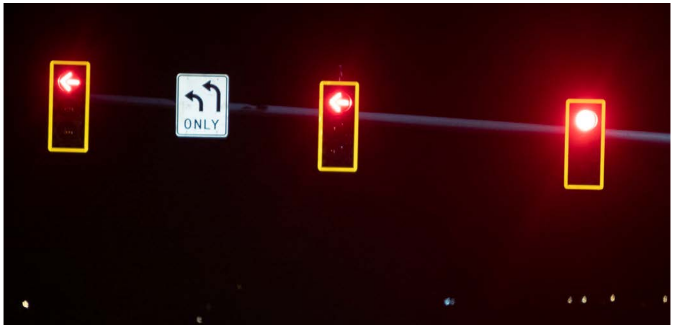
Figure 3-16 Retroreflective traffic signal backplates ( source )
