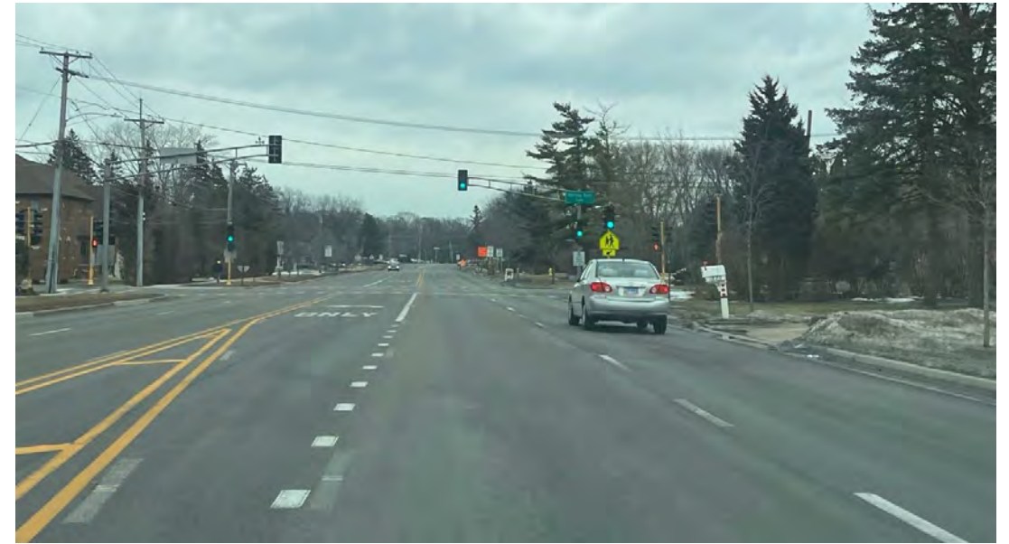
Euclid Ave & Burning Bush Ln (After Construction)
