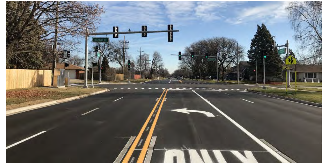
Dempster/Thacker Street & Marshall Drive (After Construction)
