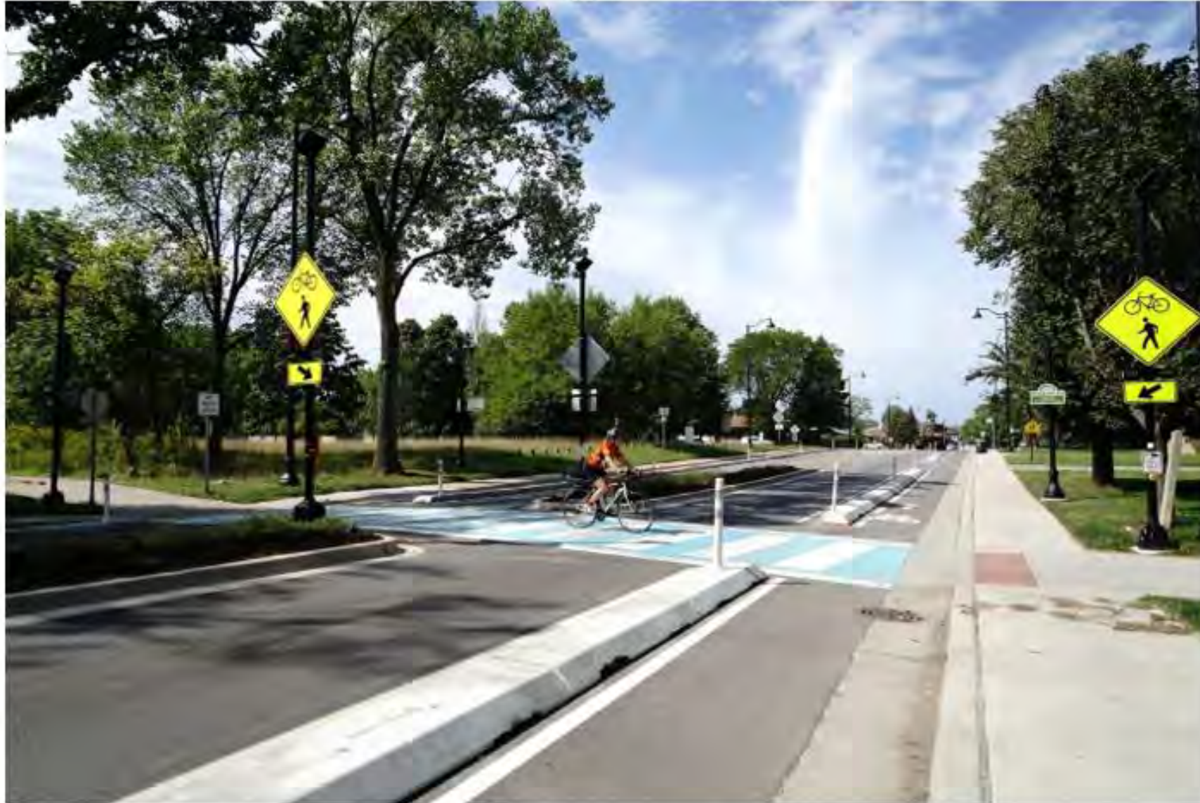
Figure 19. A recently completed road diet in Niles has improved safety by reducing travel lanes and adding features that support lower speeds.
