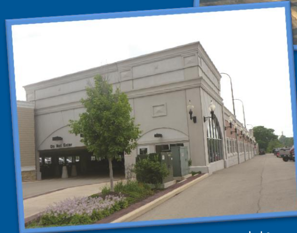
Parking deck built to accommodate future additional levels
