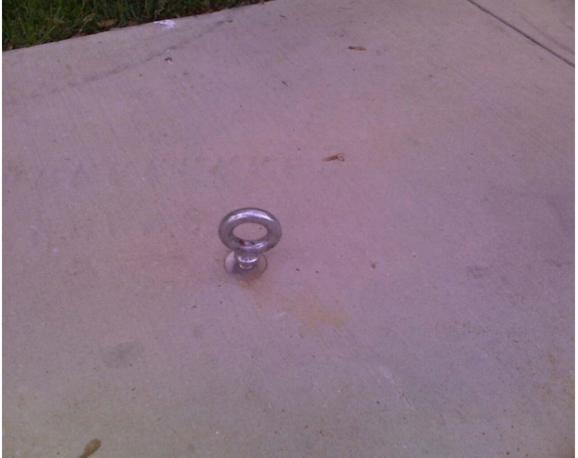
Figure 4. Cement threaded anchor (with removable hook).
