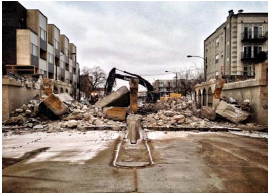
Western Avenue Viaduct demolition
