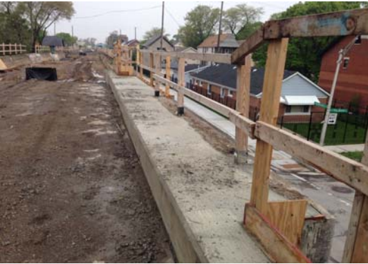
Backfilled portion of trail with new parapet curb
