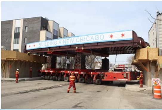
Ashland Avenue Bridge move to Western
