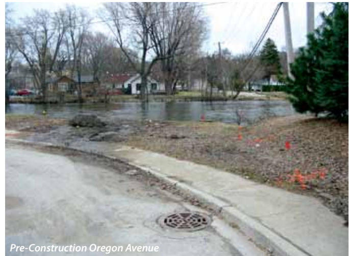
Figure 8: Village of West Dundee’s Bioretention Facilities
