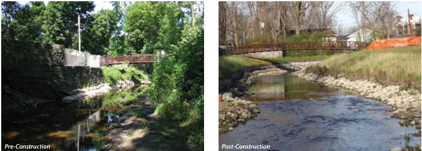
Figure 5: Buffalo Creek Streambank Stabilization Project Site
