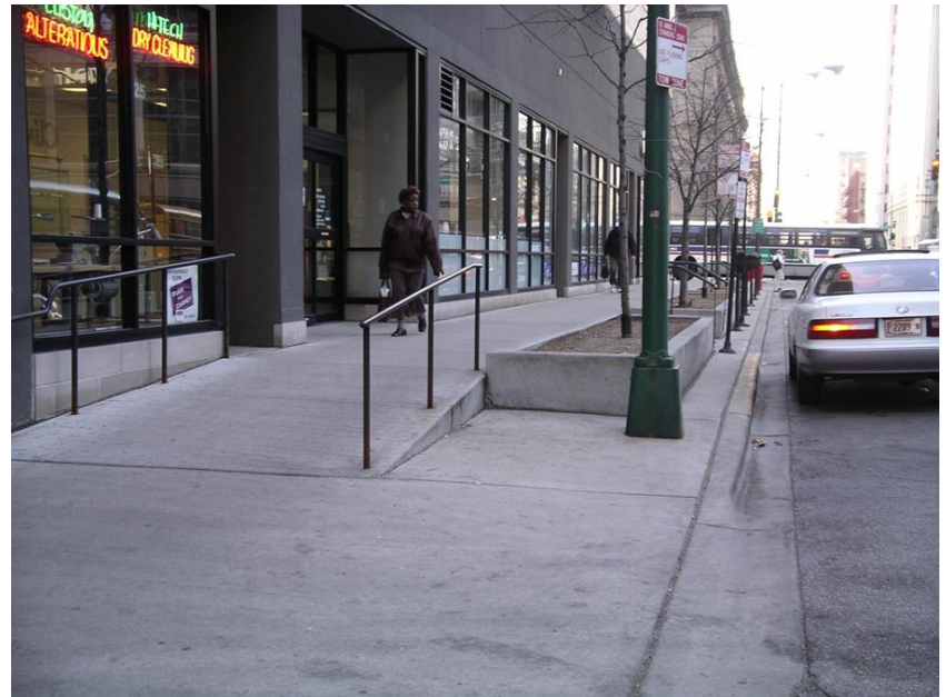
A recent accessibility improvement in Chicago
