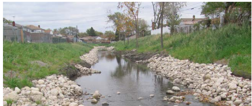
Section 319 streambank restoration project in Silver Creek in Melrose Park, IL. Photo Source: ENCAP, Inc.
