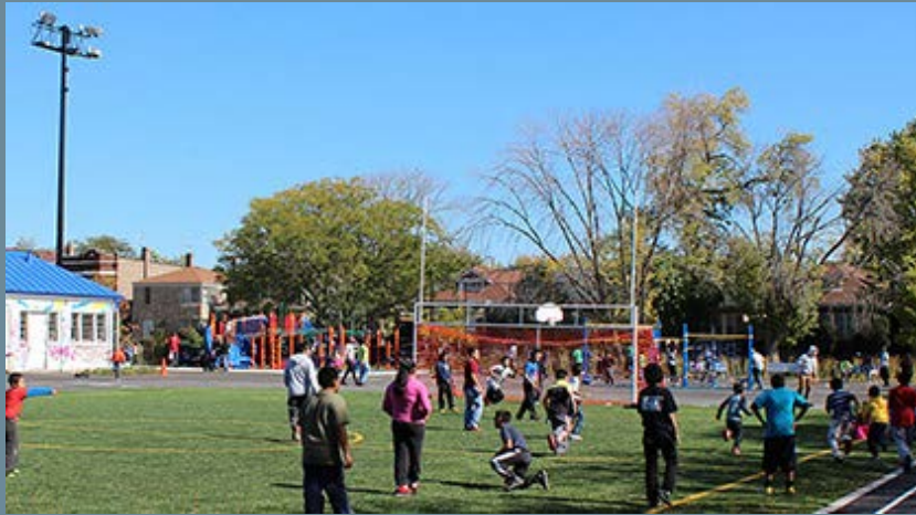
A blacktop playground was converted to a multipurpose green space and track at Morrill Math & Science School in Chicago. Drainage benefits were a part of the project.
